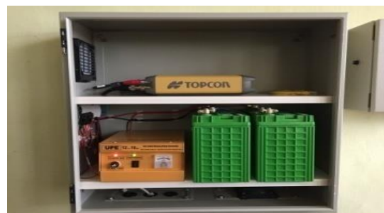
Figure 5: Base Stations and its components
